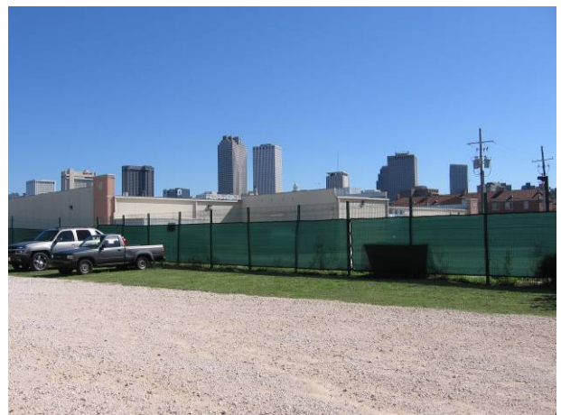
Image 3.2.1h. This site boundary was screened. Not all sites had screening – it seemed to depend on which firm had been contracted to do the site installation.
