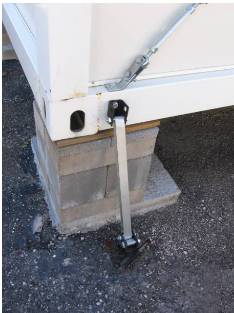
Image 3.3.1k. Anchor strap for panelized unit.
