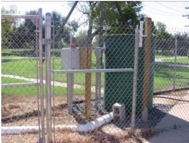
Image 3.2.2e. Fenced off water treatment area.
