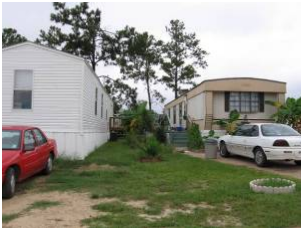
Image 3.2.1a. Commercial site with FEMA unit installed next to an existing unit.
