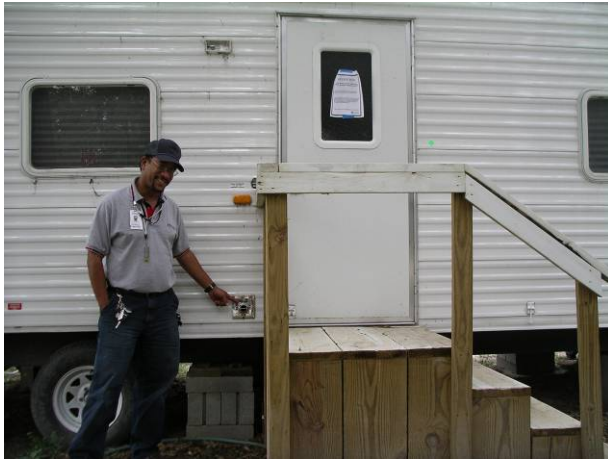
Image 3.3.3e. Some travel trailers have heat vent too close to wood stairs.
