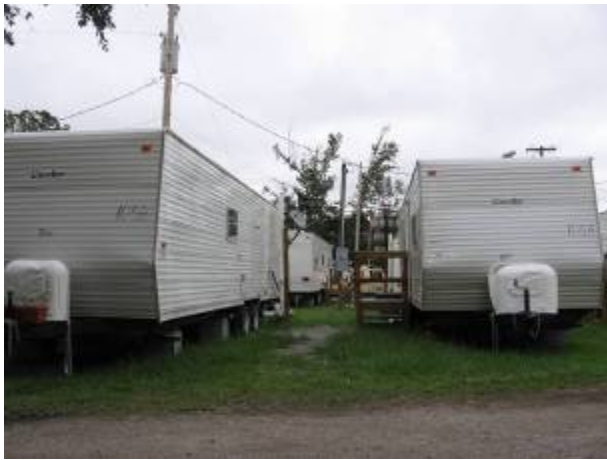
Image 3.2.1c. Spacing between units was less than 12 feet. Entrances face the back of another unit. Path to entrance is dirt/gravel which is a problem during wet conditions.
