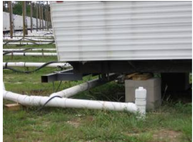
Image 3.2.2b. Detail of above ground utilities. There is no fencing around the utilities.
