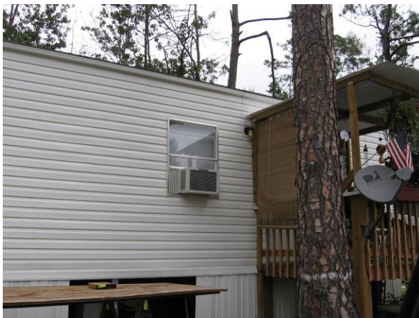
Image 3.3.3c. Window unit added to Park model.
