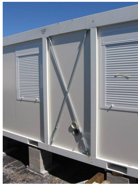
Image 3.3.1l. Panelized units were built to be stacked and are resistant to high wind conditions. Notice fresh air intake with cap.
