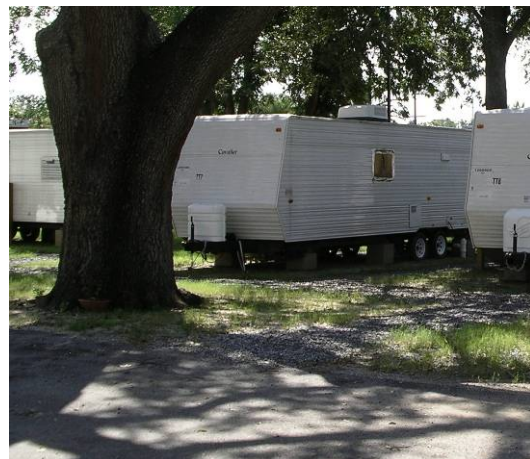
Image 3.3.3d. Roof mounted AC replaced but window still has plywood from temporary smaller AC unit.
